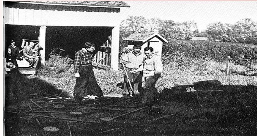
The Construction Situation
